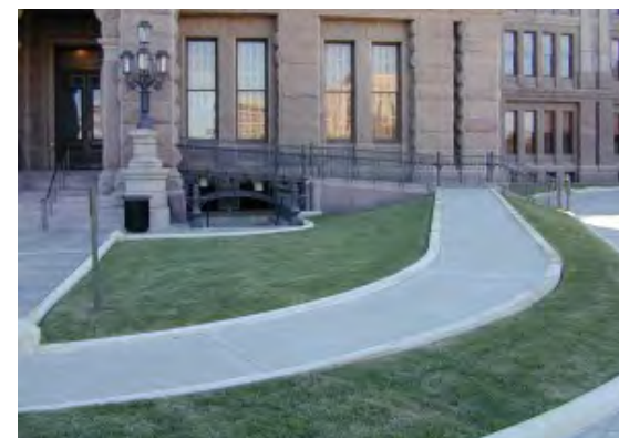
A graded path and ramp along the façade were added to improve accessibility while assuring sensitivity to the historic character of the building.
