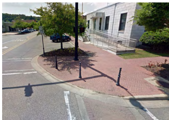
Curb extensions at corners create more pedestrian space and shorten crosswalk distance.
