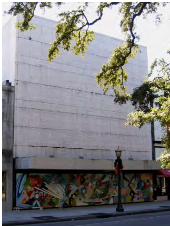
The upper portion of many historic building facades were covered in an attempt to either modernize them or stabilize deteriorating façade elements.
