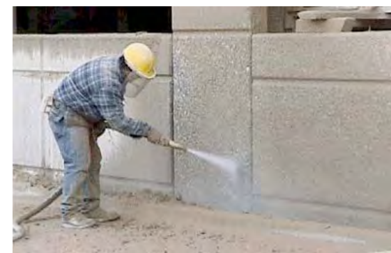
Pressure washing and particle blasting can damage or cause deterioration in wood and masonry.
