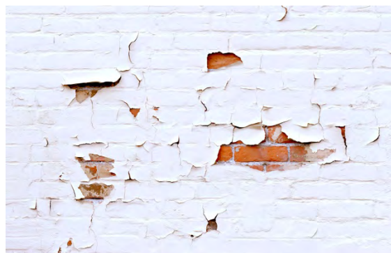
In addition to changing the character of a historic building, painting brick hides mortar problems and requires repainting over time as the paint finish deteriorates.
