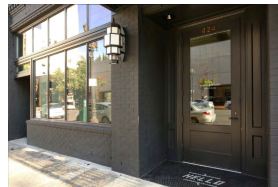
Recessed entrances allow the door to swing outward without encroaching into pedestrian space along the sidewalk.
